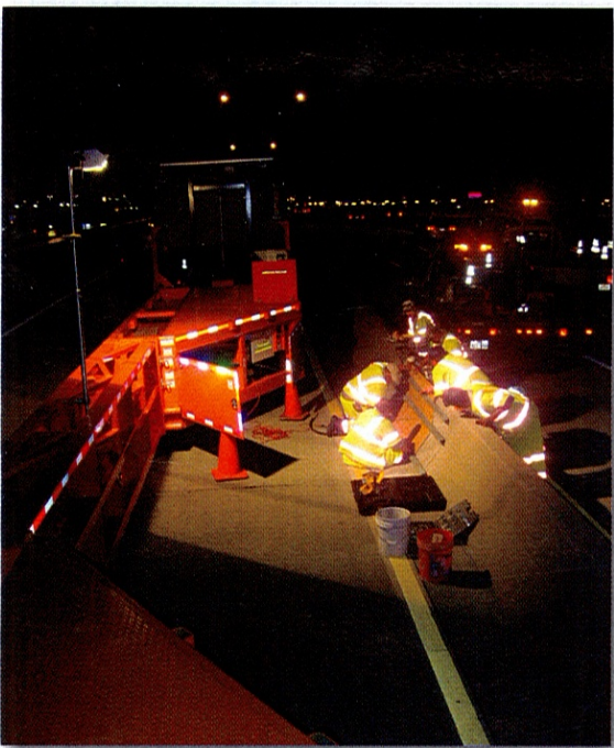
The MBT-1 Mobile Barriers Trailer provides a well lit work area as well as a source of electrical power for the temporary highway maintenance job site while completely blocking any traffic hazard from the road.
