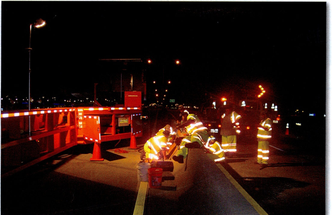
ANSI Class 2 or Class 3 high-visibility safety apparel is now required for all workers exposed to traffic or to construction equipment while working within the rights of way of federal-aid highways.
